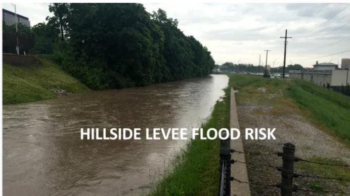
There are two functions for the Hillside Levee – allow backflow from high water on the Missouri River and to prevent flash floods from rainfall above the City.
