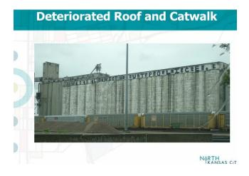
Significant decay and unsafe conditions are present at these old silos at 1400 Nodaway, located between the railroad tracks which parallel Bedford Road. Although complete demolition is probably inevitable and has been included in the current year budget, notice was given that some unsafe conditions will be repaired and/or made inaccessible to individuals who have been in the buildings. There is evidence of occasional occupancy because of graffiti that has been painted on some of the structures.
